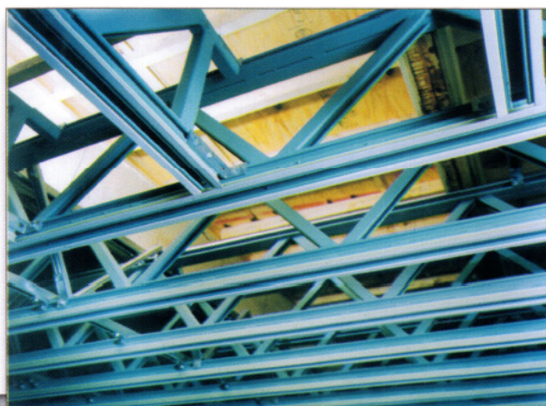
Roof Truss / Ceiling Grid
