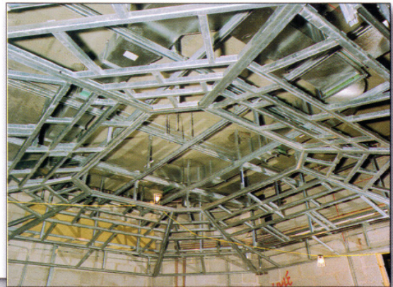
Structural Ceiling of Complex Design
